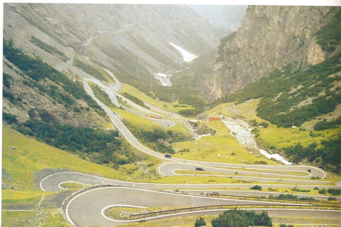
Approach from Bormio (south ramp) to the Stifser Joch.
