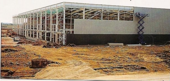
The new Triumph factory is starting to take shape.
